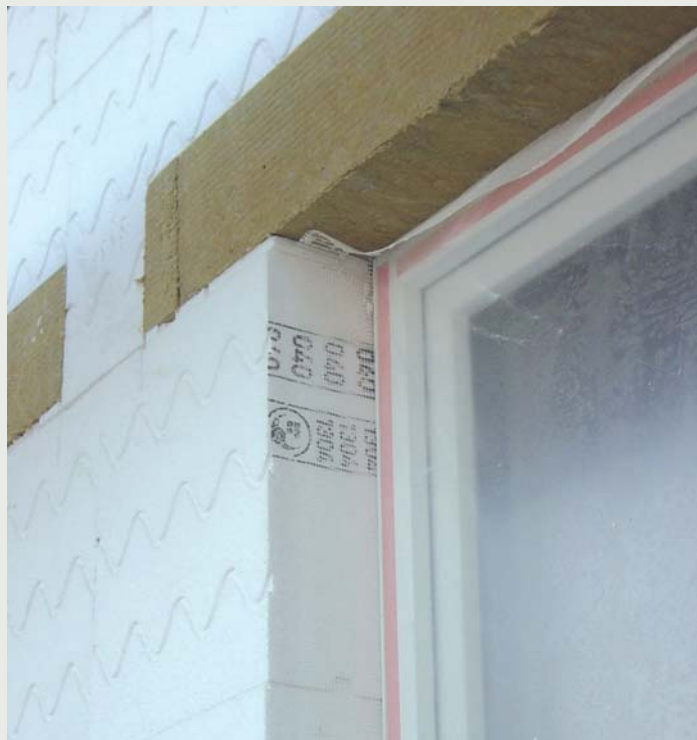
A blower door test (above left) is a mandatory requirement for all certified passive houses; insulation detail (above right) around a well insulated window in a passive house
